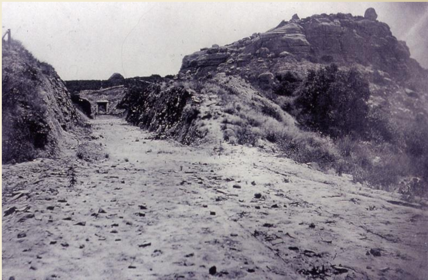
West side of Tunnel 28 looking east
